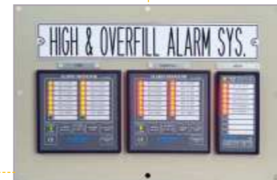
High & Overfill Alarm Unit
