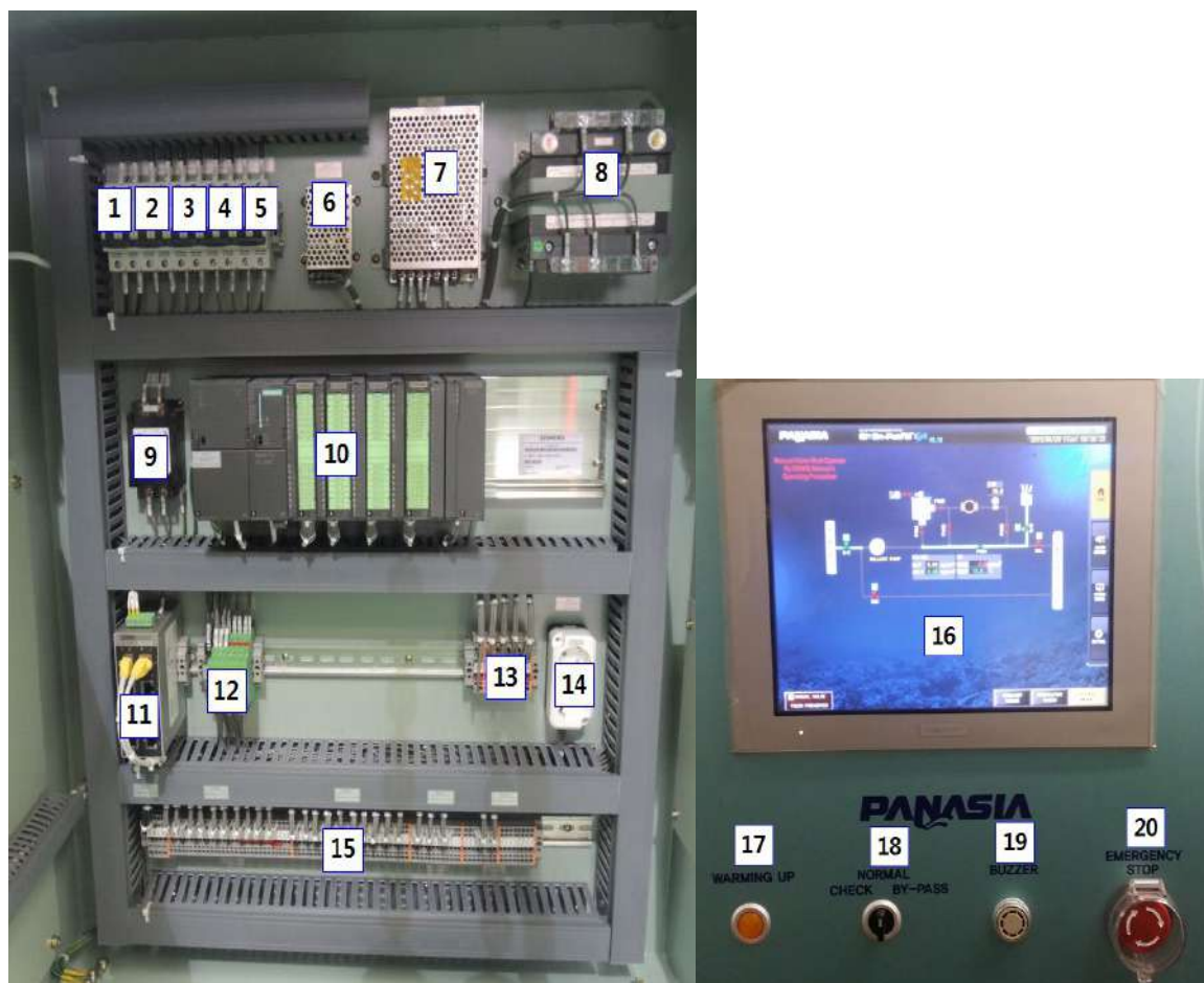
Figure 7.34 Components of the control panel
